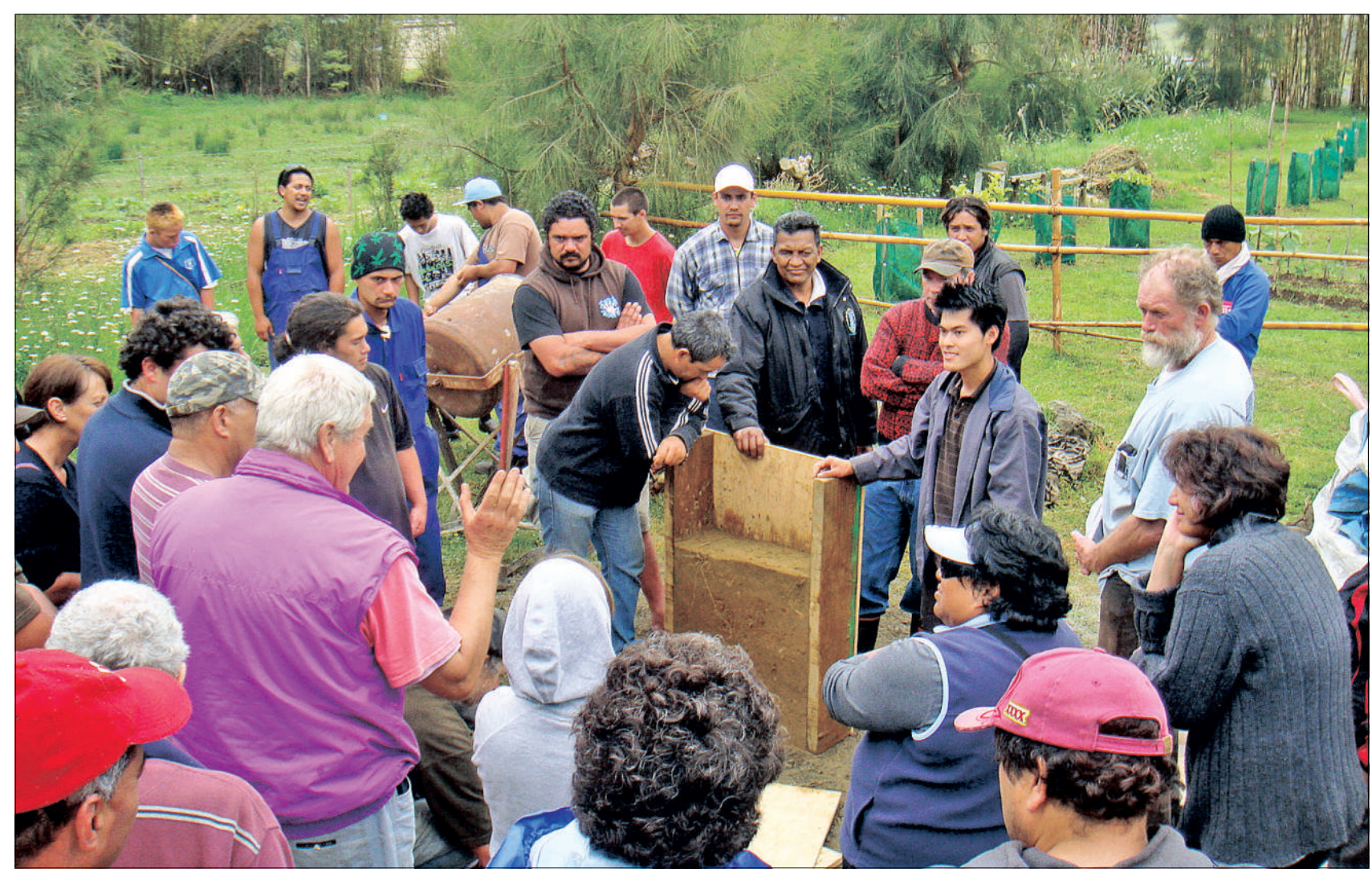
THIS IS HOW you do it — lessons in building with rammed earth got under way at Ahipara yesterday, and will continue for the rest of the week. Photo supplied.
